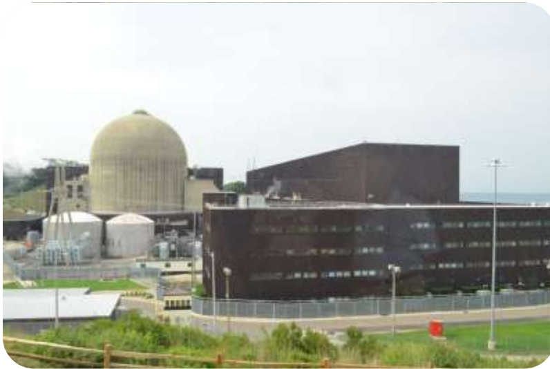
Participants and Lecturers of this course visited the DC Nuclear Power Plant in Bridgman, MI Photo Credit: Kun K., Argonne National Laboratory
